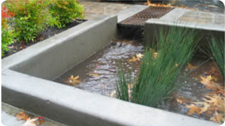
Infiltration planters with curb cut and trench drain
